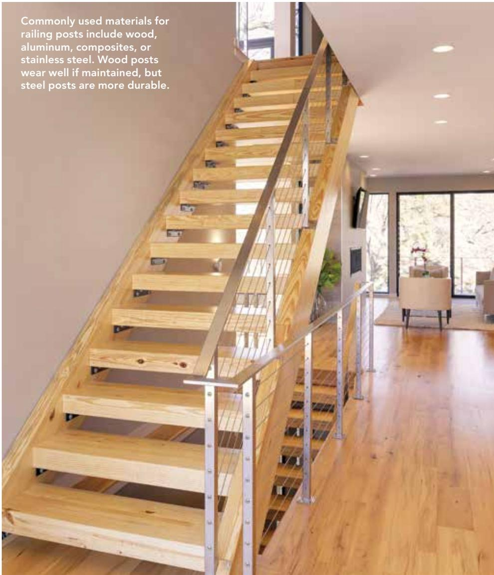
to length on-site, stainless steel railings must be custom fabricated before they can be installed.
