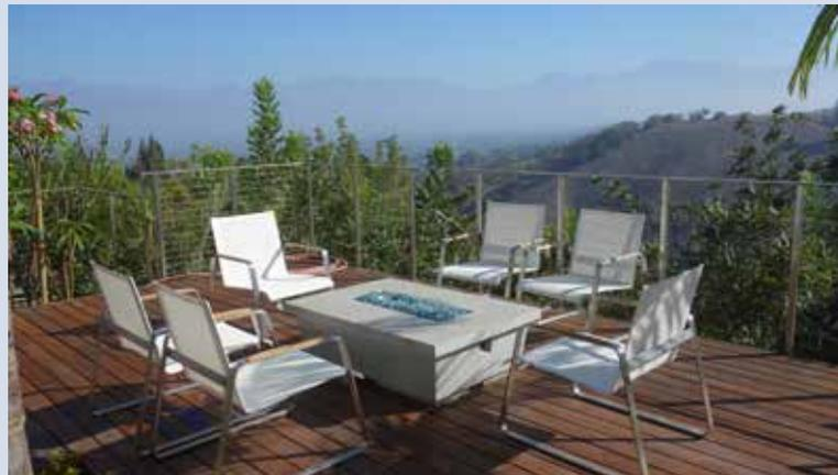
**Steel has many advantages over aluminum, including strength and longevity. In exterior applications, stainless steel can outlast aluminum by decades with little maintenance. This image shows stainless steel railing configured with a side mount post, cable rail, and flat top rail.**
