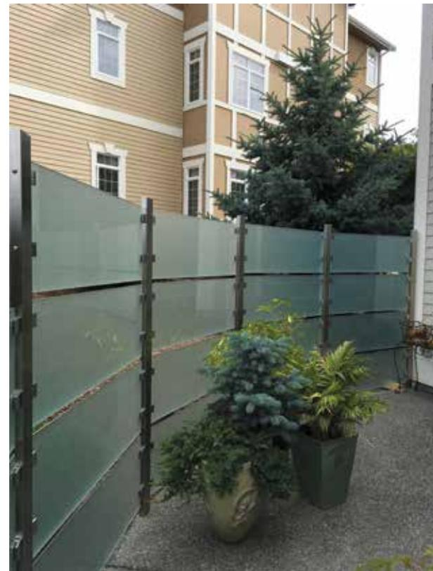
Glass as an infill material can help provide a sense of privacy, security, and also, when clear, open up visibility for occupants.
