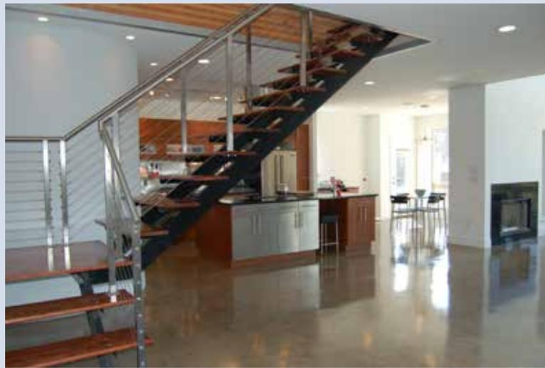
**Aluminum posts and handrails tend to be much thicker than their stainless steel counterparts. A “strength-equivalent” stainless steel post is 50 percent thinner than an aluminum post, which can help open up interior spaces and create a more contemporary design.**
