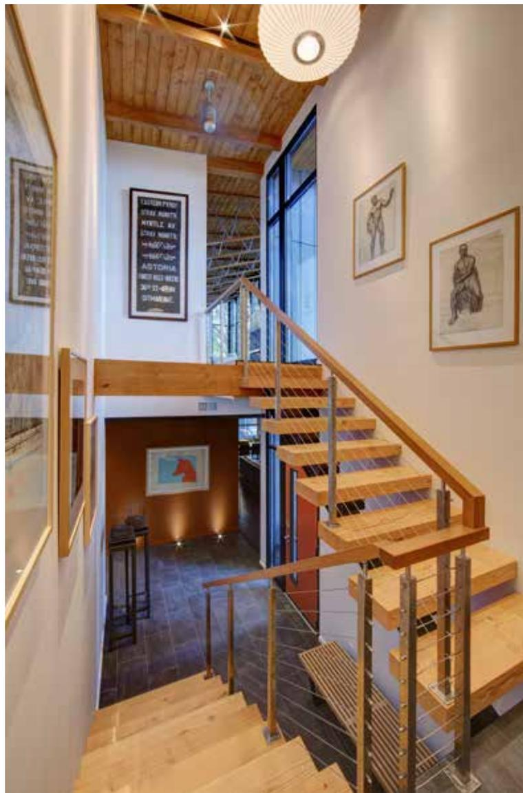
One of the main benefits of prefabricated ornamental railing is that it removes the need for TIG welding. TIG welding can present some possible safety hazards that are best managed in the controlled environment of the manufacturing plant rather than in a residential or job-site environment.
